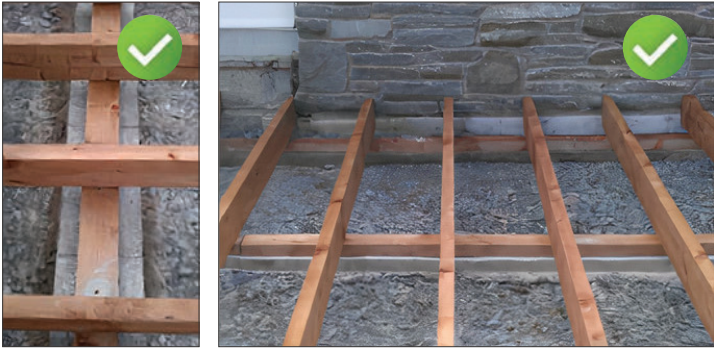
Bridging supports can be put in as required.
