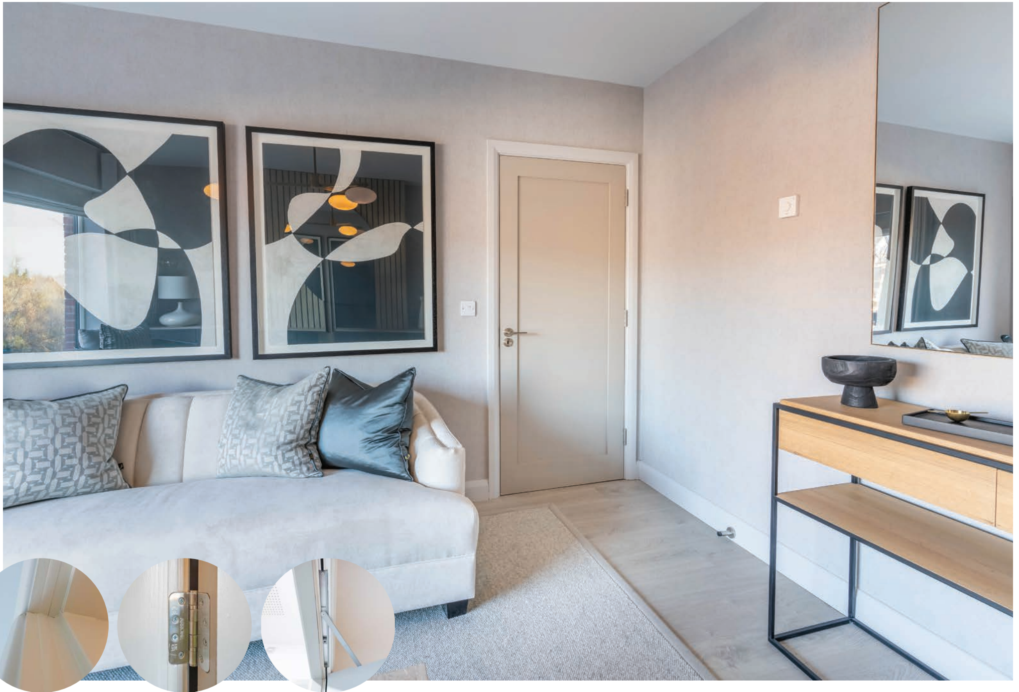
Fire Door Safety Features: Intumescent Fire Seal, Fire Rated Hinges and Concealed closer.
