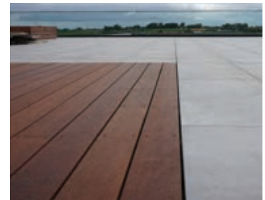
Pedestals give great flexibility for installations and make it easy to allow decking and paving to be installed easily in the same area.
